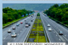
6 LANE NATIONAL HIGHWAY
